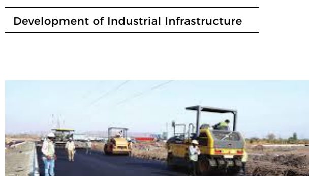
DMIC VIKRAM UDYOGPURI LTD. Infrastructure Development Works
